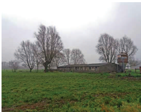
Figure 5. Weathered grain silo and shed (© Timon Lamoot)
